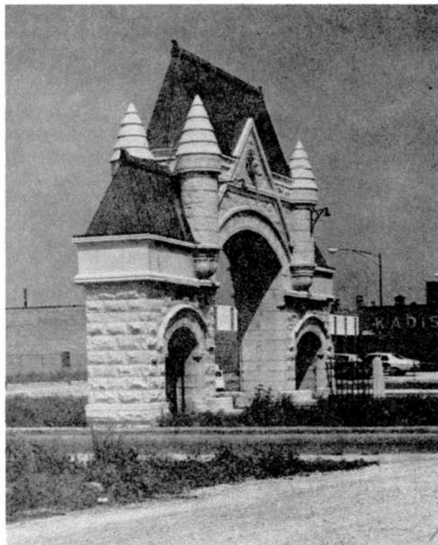
Southern wing (left) refinished with rusticated blocks and trim bands cut from the demolished guardhouse. (Barbara Crane, photographer)
